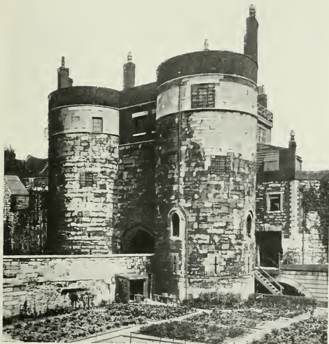
56. The Byward Tower, Tower of London.
